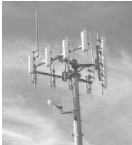
Figure 16.5 Sectorized base-station antenna.
